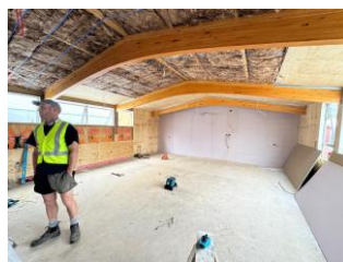
Bats are going in and some wall linings are on.
